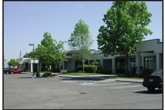
±2,727 SQ. FT. OF OFFICE SPACE FOR LEASE 346 W. GRANT LINE ROAD, TRACY $0.90/SQ. FT. NNN SUITABLE FOR CALL CENTER OR OTHER BACK OFFICE USES
