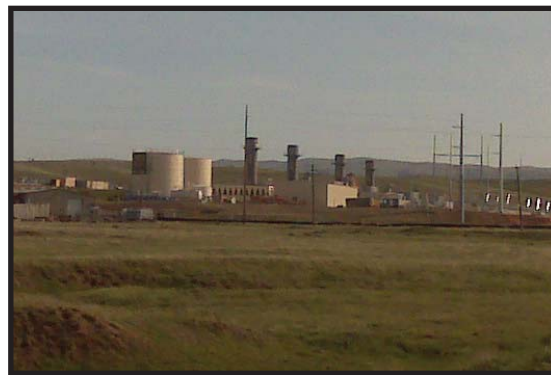
Mariposa Energy Project
